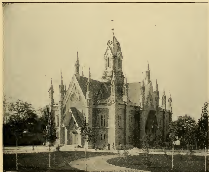
THE ASSEMBLY HALL.
